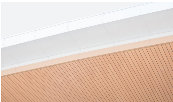
Left: Standard Timber Cladding installed as a ceiling feature.
