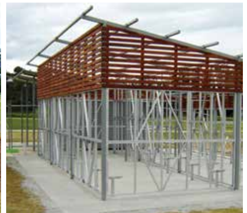
STEEL FRAMEWORK AND WALLS ON-SLAB
