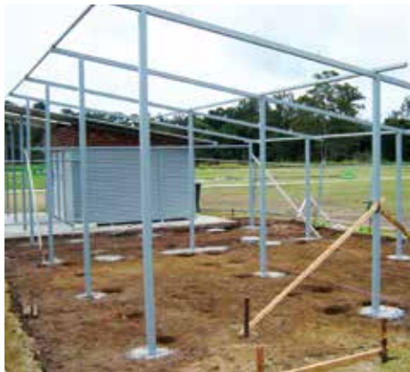
STEEL FRAMEWORK WITH FOOTINGS
