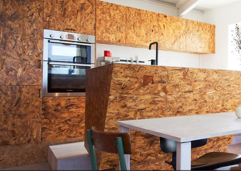
Strong, stable and more sustainable, oriented strand board (OSB) is a greener alternative to plywood. Timeless timber colour and properties with an abstract flair - OSB is ideal for internal wall linings, cladding, shop fitting, decorative paneling, cabinetry, office fitouts and displays.
