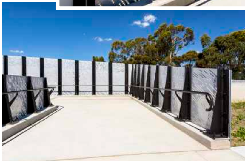
Lakes Boulevard Shared Use Pathway, Mernda, VIC Supplied and Installed by Stoddart
