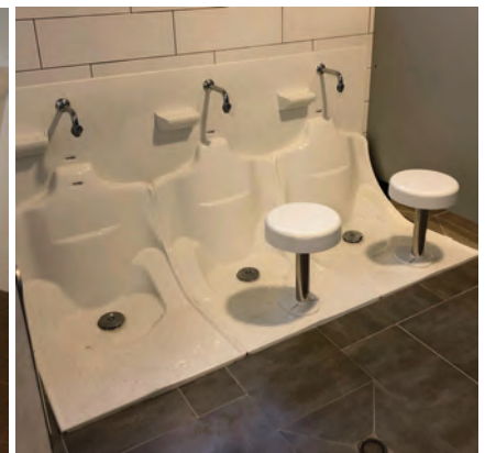
WM MODULAR SHOWING A DISABLED UNIT FOR WHEELCHAIR ACCESS
