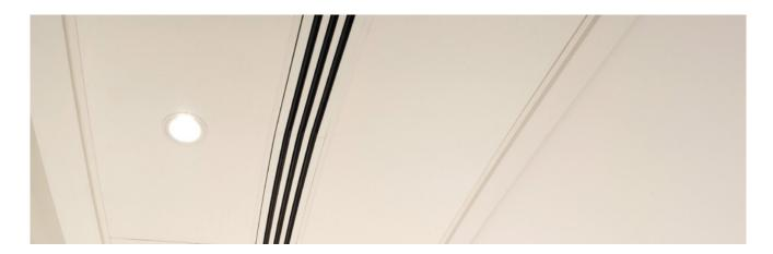
A tile-only system, SAS320 has no gridwork, reducing costs and allowing for quick and simple installations. The system is suspended from edge trims or other suitable features such as lights or grilles. Intended for corridor and plasterboard surround applications, SAS320 is ideal for residential and commercial sectors with targeted acoustic demands. Tiles can be of any size to suit most building modules and trimmed for improved aesthetics across undulating walls.
