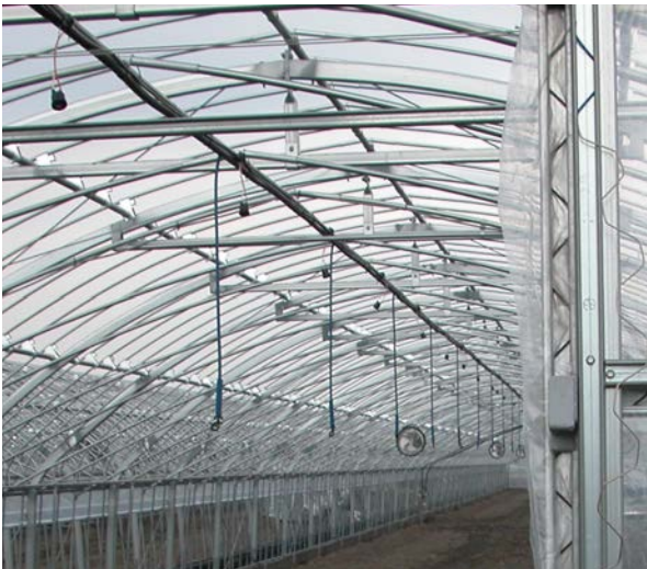
ZAM ® framing on greenhouse
